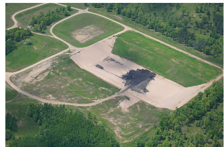
Top: Niagara Landfill operations Bottom: Aerial view of Niagara Landfill
